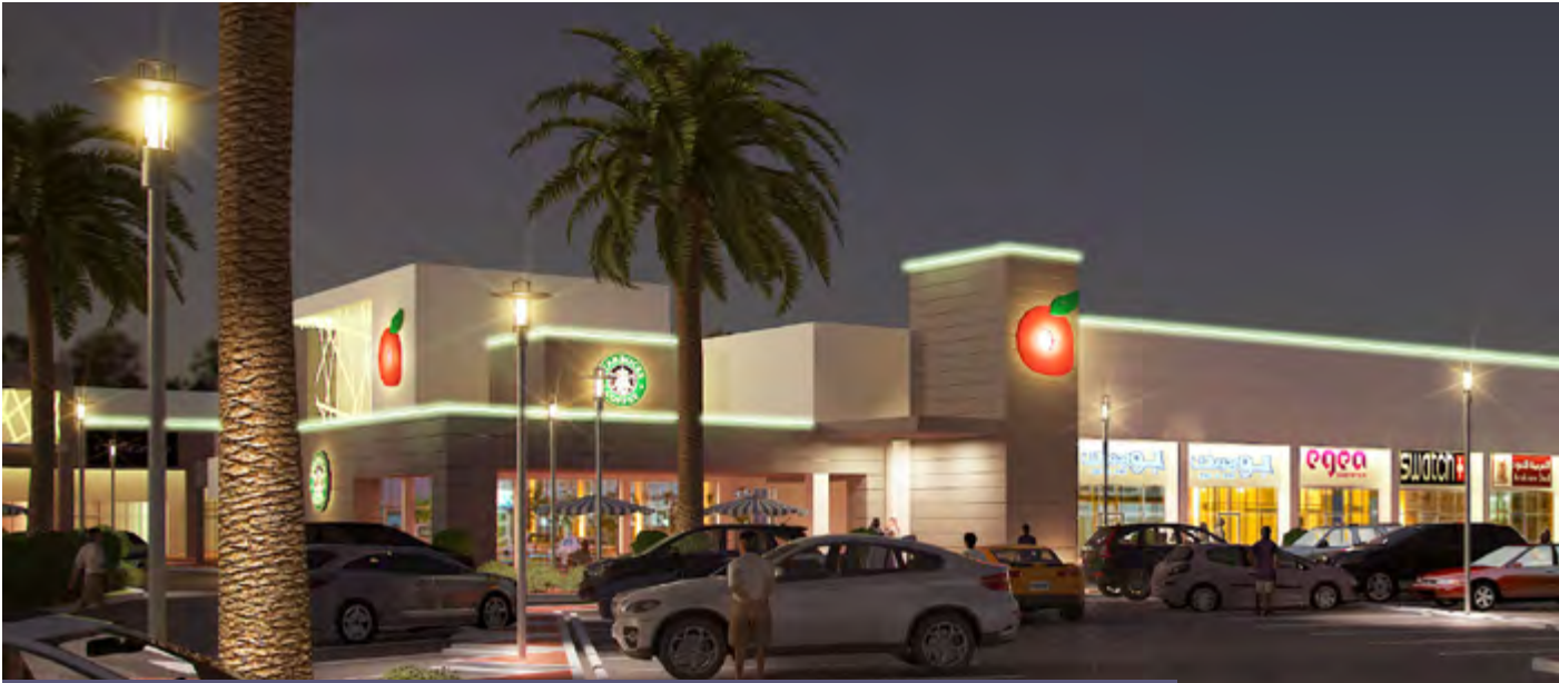
Renovation of Al-Takhassusi Plaza
