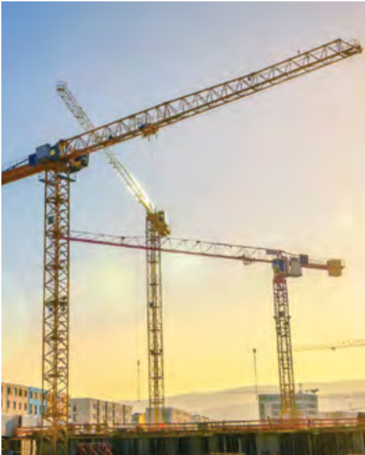
Expansion of Makarem Riyadh Airport Hotel
